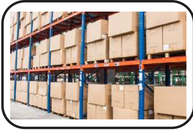
Selective Pallet Racking
